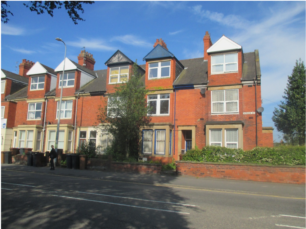
Photograph of front elevation
